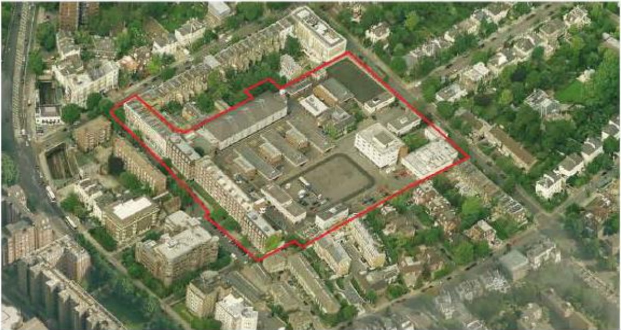
Aerial view of site – from the applicants submission (prior to any demolition on site)
